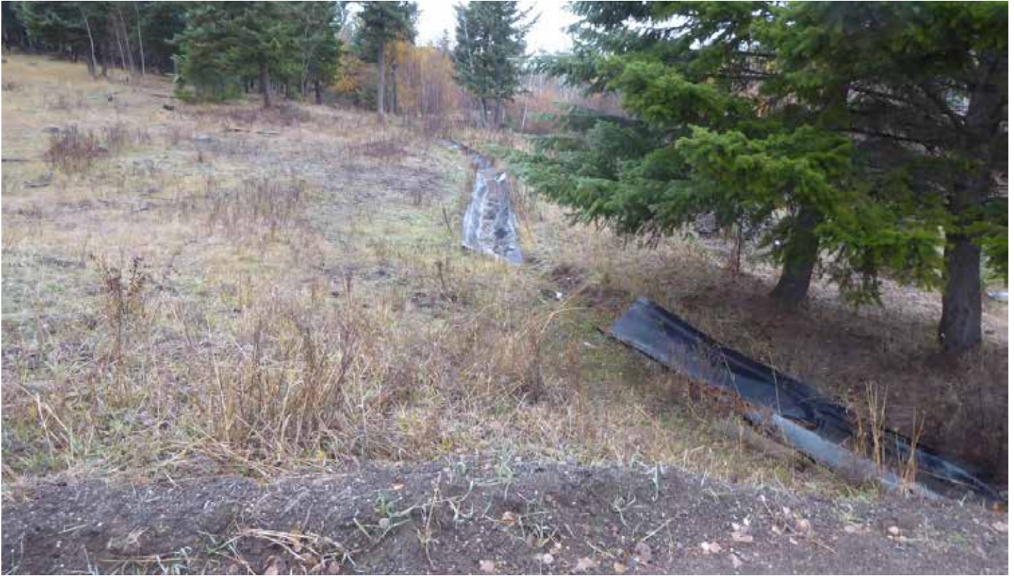
A long-abandoned flume on the west side of the Campbell Range Road. Water flowed down the flume towards the road from a small lake about 800 metres to the west.
