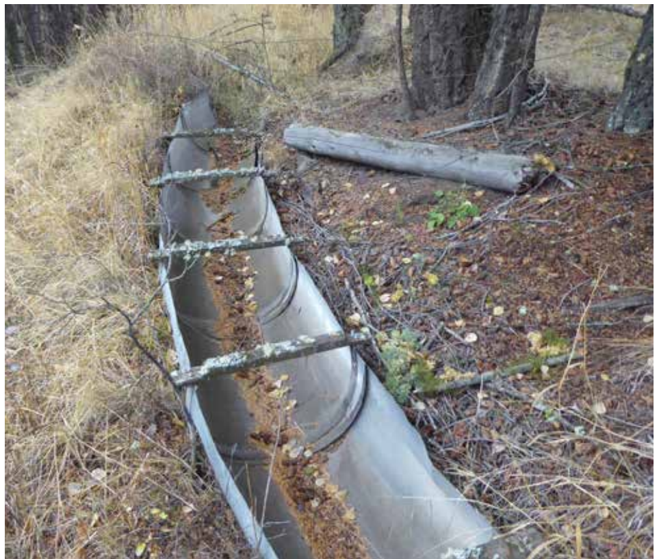
A continuation of the same long-abandoned flume but on the east side of the Campbell Range Road. The water went through a culvert under the road.
